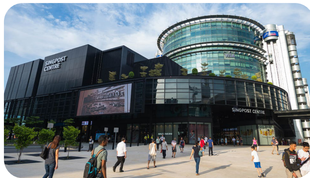
SingPost Centre (Commercial) achieved BCA Green Mark Gold Plus award
